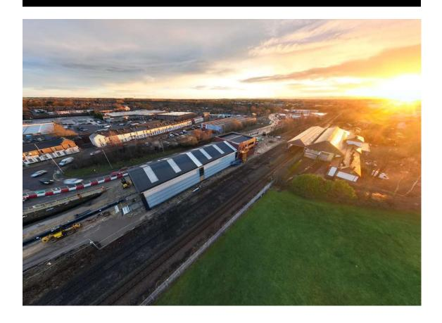
As the sun rises on a new year, we look forward to moving into our new home. Plans are afoot for the move in May. On the new building, the windows are fitted around the offices and viewing platform. The internal rails are now set into the floor of the main shed, and outside the inspection pit has been sunk into the ground. The Trust has sourced rails and sleepers at concessionary rates as the opportunities arose over the last couple of years, however they were unfortunately not donated gratis.
